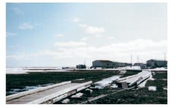
Fig. 15.14. Boardwalk damaged by storm surge flooding, Kipnuk, Alaska (photo by Mike Marcaurele).
