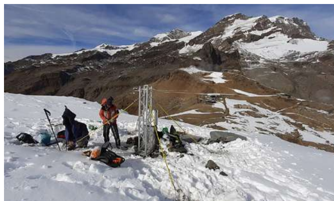
Fig. 22. Maintenance of the permafrost station at Salati Pass (ARPA Piemonte).
