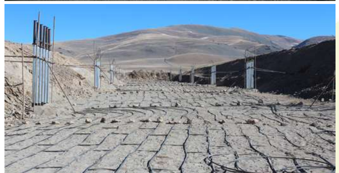
Fig. 32. Thermosyphons installed along a roadway to prevent thawing permafrost and settlement of the road surface.
