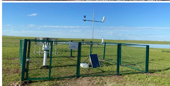
Fig. 16. Installation of soil temperature and moisture sensors in the active layer (top) at the new meteorological and active layer hydrothermal site in Bagannuur, Mongolia (bottom).
