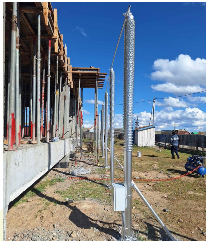
Fig. 37. Foundation with open crawl space and inclined thermosyphons in Arbulag soum, Hovsgol province, Northern Mongolia.
