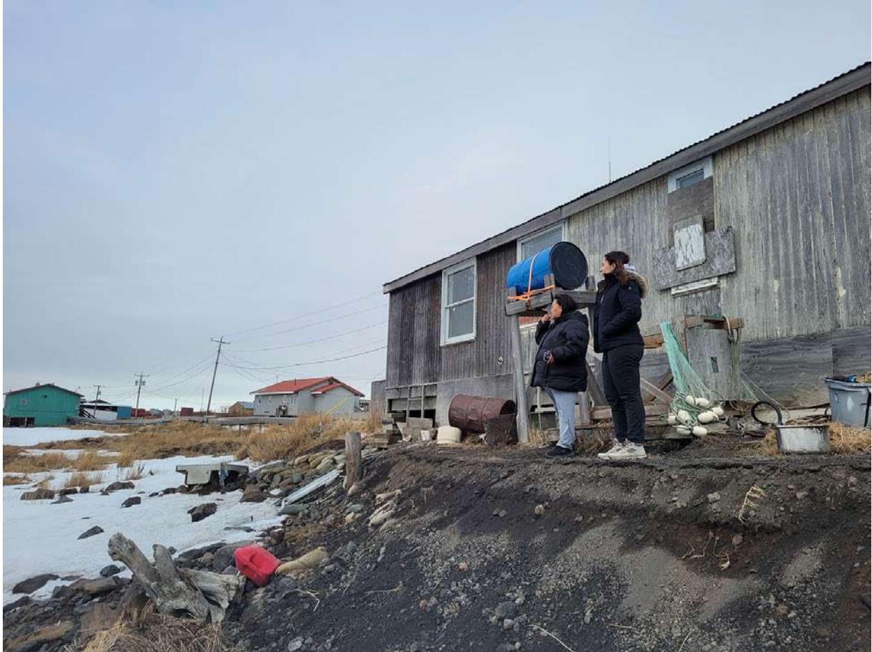
Fig. 2. Coastal erosion monitoring in Golovin, Alaska, is conducted by local observers documenting shoreline change as part of regional monitoring efforts. Such observations provide critical information for understanding climate impacts in vulnerable communities. Credit: Hannah-Marie Ladd.
